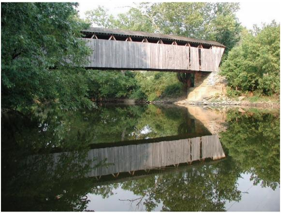
The Switzer Covered Bridge once carried Ky. 1262 across North Elkhorn Creek at Switzer in eastern Franklin County. It is a 120 foot long Howe truss design built in 1855 and restored in 1906 and again in 1990. On March 1, 1997 the bridge was washed away in a flood and was restored in 1998. Located approximately 0.1 miles east of Ky. 1689 (Switzer Road) on Ky. 1262. The bridge is on the north side of Ky. 1262 over North Elkhorn Creek. Photo by Brandon Nuttall, Kentucky Geological Survey.
